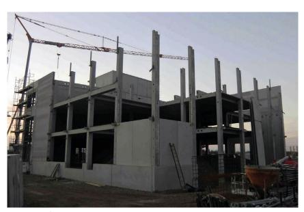
Figure 1 Reinforced steel supports as natural down conductors
